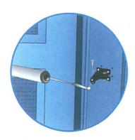
Detach screen door piston and bracket from door frame.
